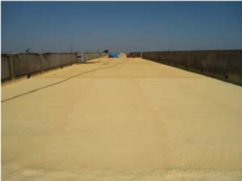
FIGURE 11 OVERDECK SPRAYED RIGID INSULATION
