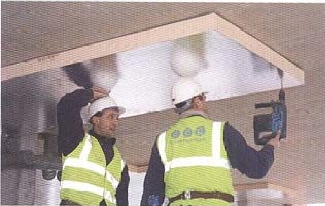
FIGURE 13: UNDER DECK RIGID INSULATION
