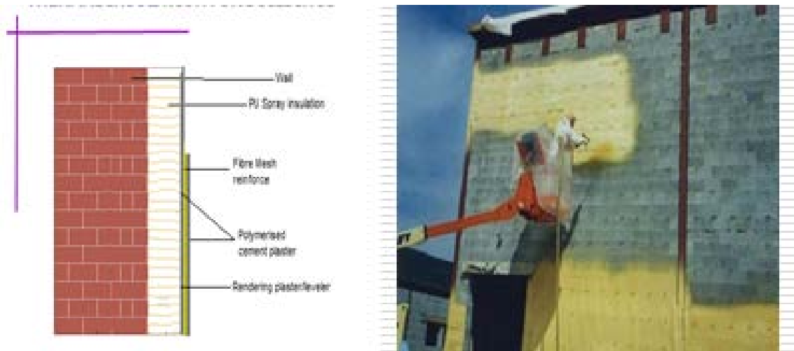
FIGURE 20: SPRAY CAST IN-SITU INSULATION
