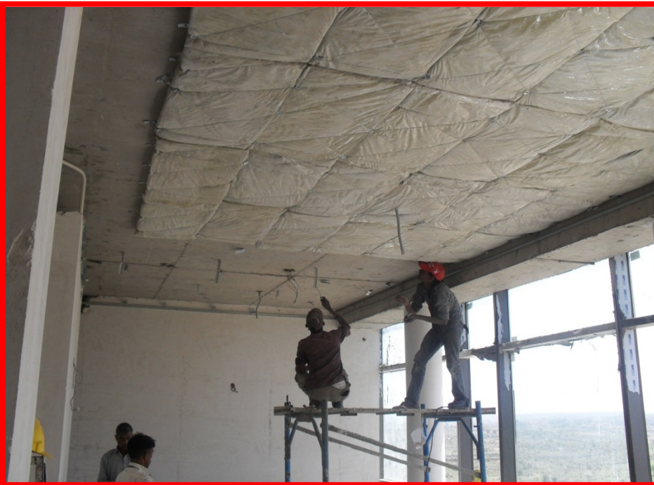
FIGURE 12 UNDER DECK FIBROUS INSULATION
