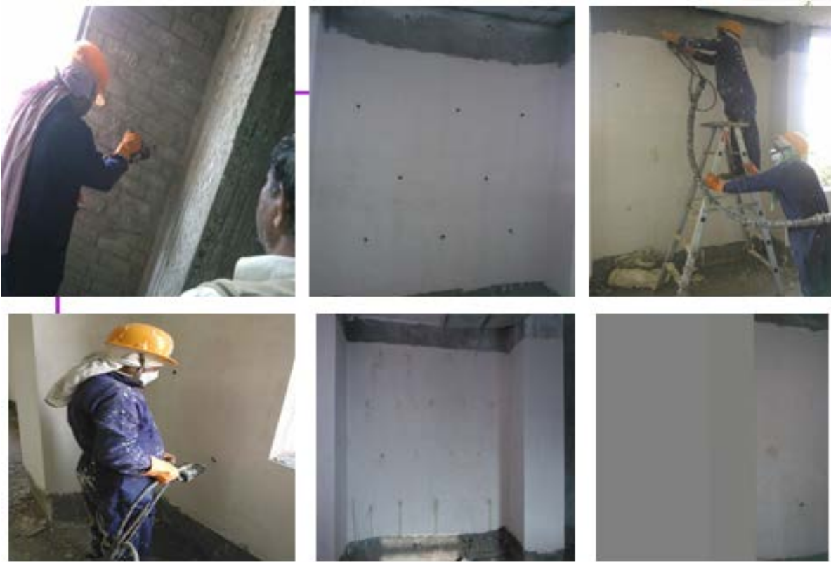
FIGURE 14: SPRAY IN-SITU INSULATION
