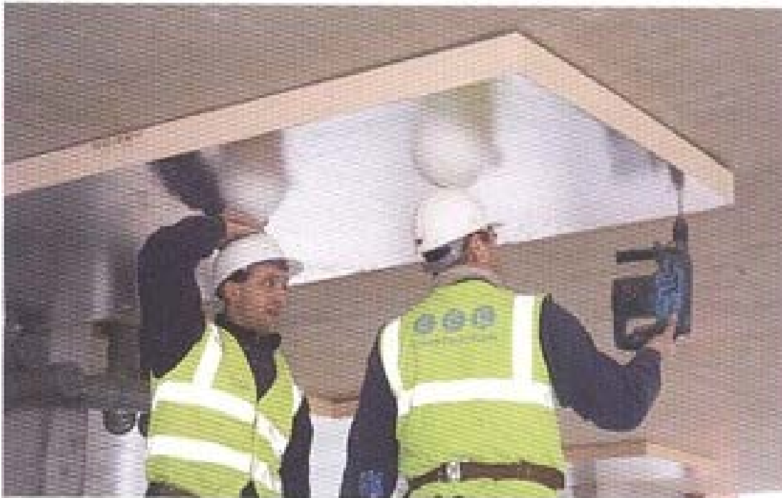
FIGURE 13: UNDER DECK RIGID INSULATION
