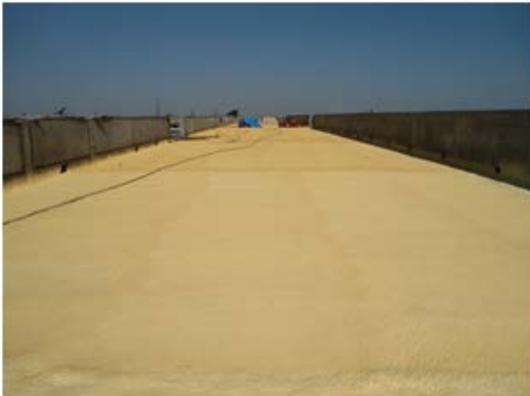
FIGURE 11 OVERDECK SPRAYED RIGID INSULATION
