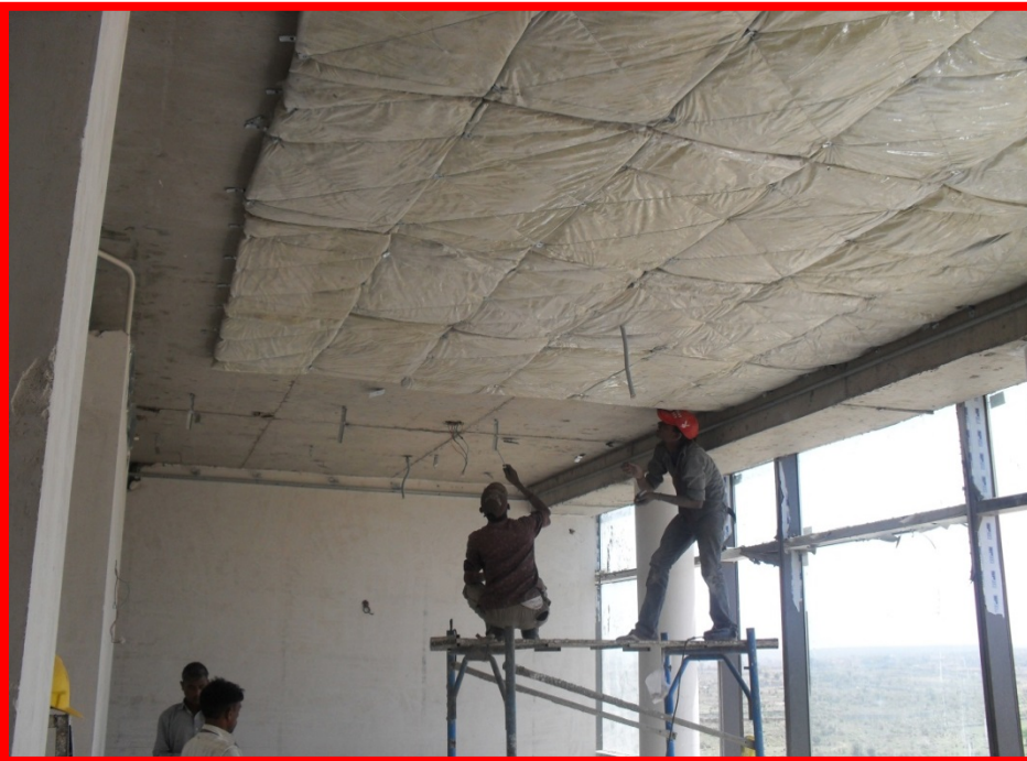
FIGURE 12 UNDER DECK FIBROUS INSULATION
